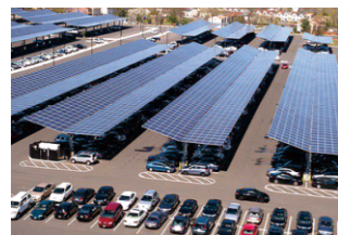
Commercial car park
