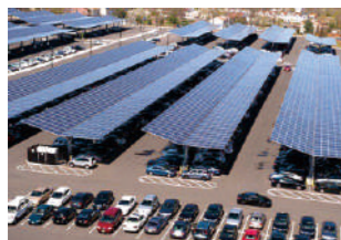
Commercial car park
